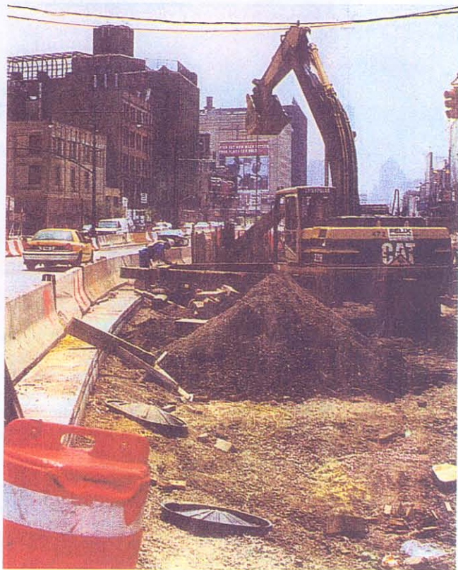
SEPARATION Barriers give more protection than barrels.
