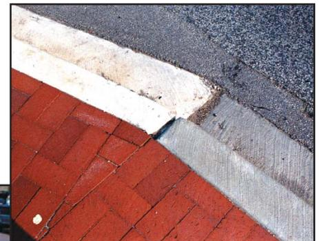
**Figures 2 and 3.** The difference between white and gray concrete can be pronounced, as seen here in a close-up of adjacent curbs of the two different colored materials. Seen from a distance, the white curb catches the eye while the gray one blends in with its surroundings. (70159, 70160)
