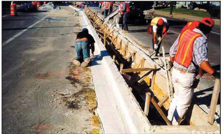
*Figure 12. Standard placing and finishing techniques are used for white cement concrete, though attention to clean tools and other equipment should be exercised. (70168)*
