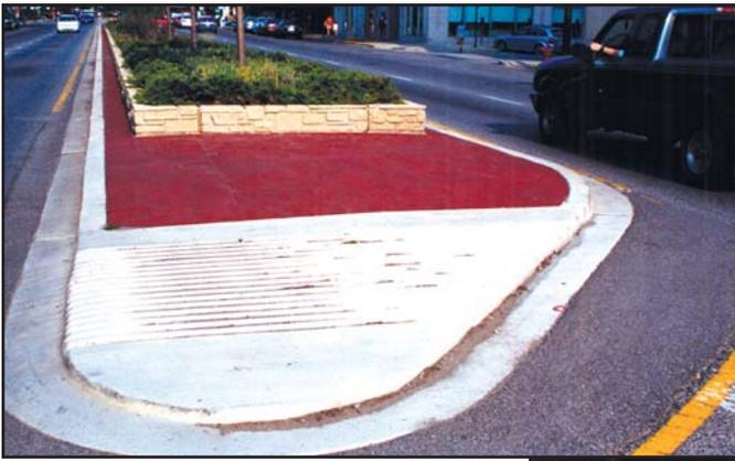
**Figure 4.** White concrete nosings channel traffic at the ends of median strips. Even with scuff marks and debris from the street, the bright white color shines through. (70161)
