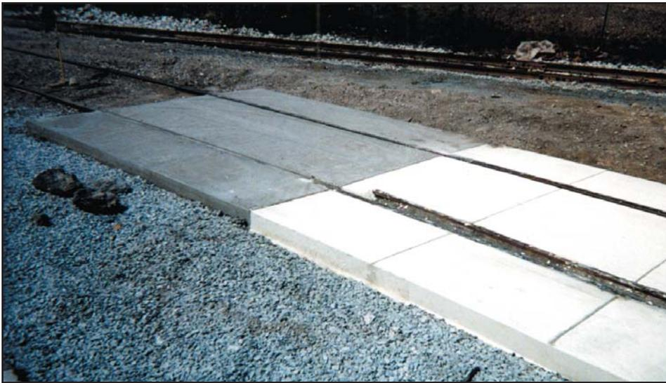
**Figure 9.** Railroad tracks that cross at grade are very dangerous. Any means of improving visibility, such as constructing crossings with white concrete, can increase safety. (70166)
