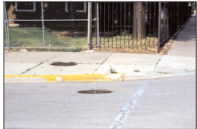
**Figures 7 and 8.** Painted walks and curbs eventually need to be repainted. This chipped and peeling yellow paint decreases a property's appearance, be it an adjacent building or a city street. (70164, 70165)
