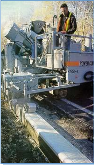
Innovative slip forming of white concrete over gray concrete
