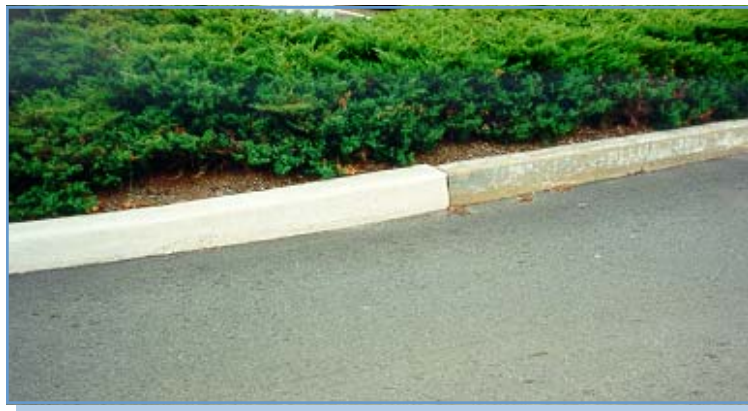
White concrete against painted concrete
