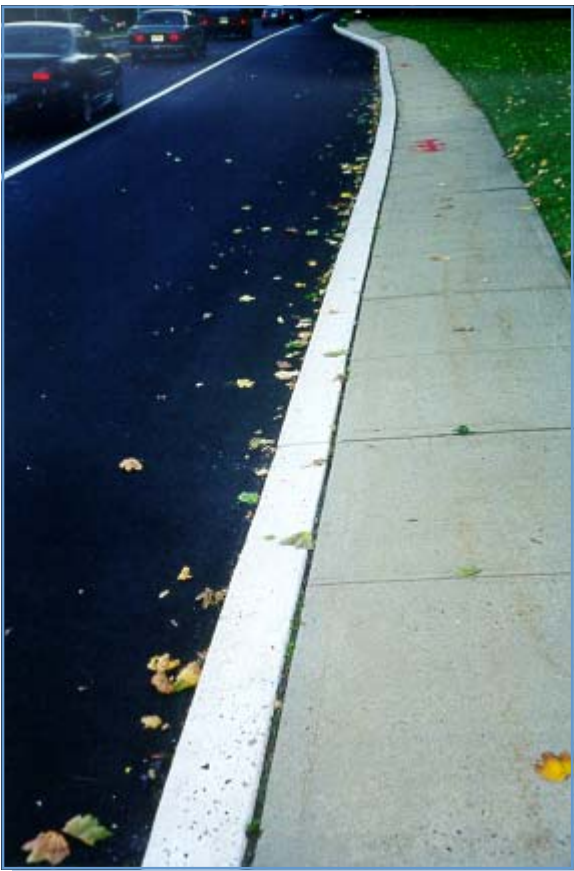
White concrete curbing is easily visible and provides safety at schools or in building unloading zones.
