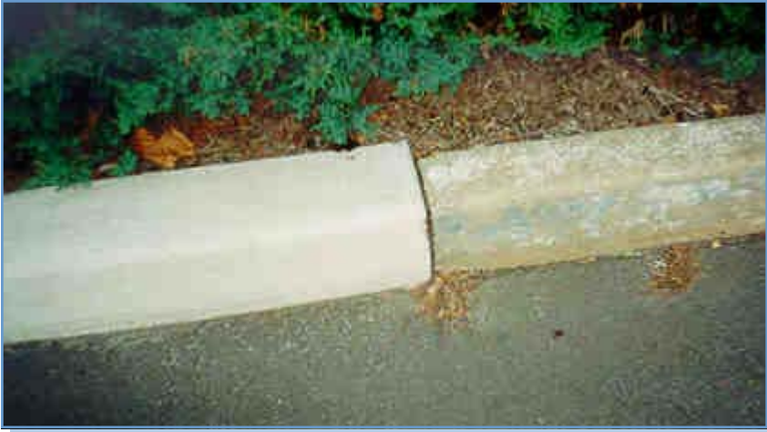
White concrete curbing or gray concrete curbing? Which is easier to see and maintain? (No painting necessary!)
