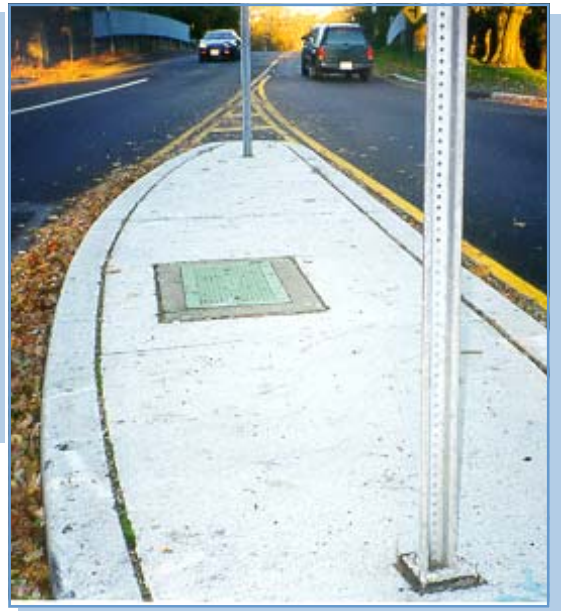
Turning lane channelizer
