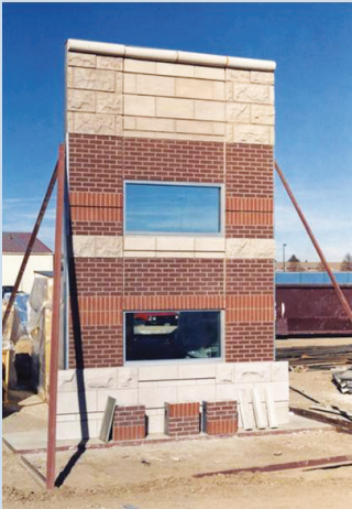
Figure 3. A sample panel, or mockup, allows owners, designers, and builders an opportunity to agree on the appearance of the wall before construction begins.
