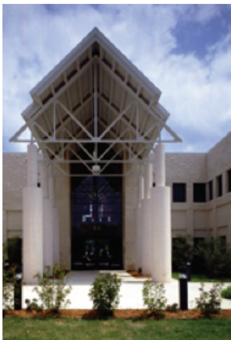
Figure 1. Visually, mortar can represent a significant portion of a masonry façade. Where a white masonry wall finish is desired, white units should be assembled with white mortars.
