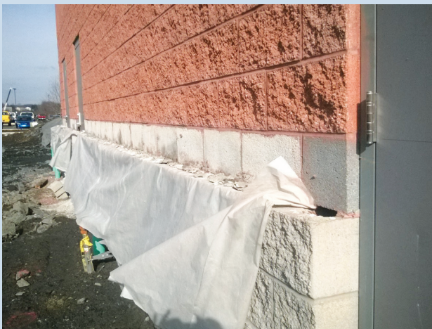
Figure 5. To prevent unwanted buildup and additional cleaning, protecting tops of walls and previously completed work is an essential best practice.
